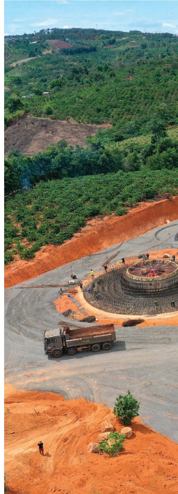
Wind farm under construction in Dak Lak, Vietnam.
