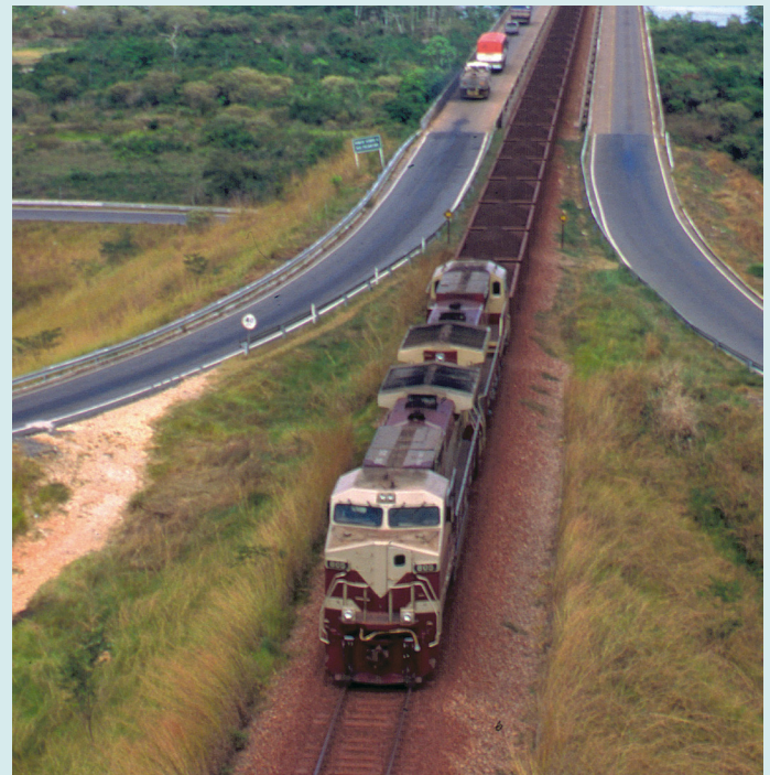
Photo: Iron ore train on the Marabá Road–Rail Bridge across the Tocantins River.
