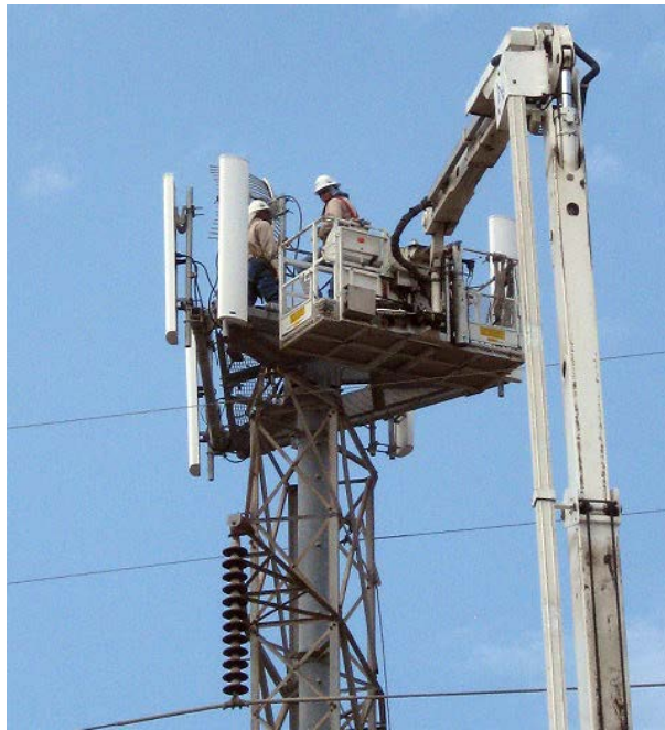
Figure 8.13: Installation of cellular antenna on electric transmission tower
