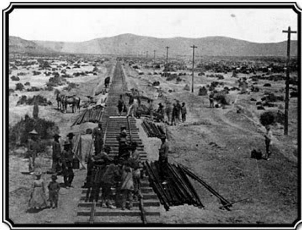
Figure 8.49: Simultaneous construction of transcontinental railroad and adjacent telegraph poles in 1868 293
