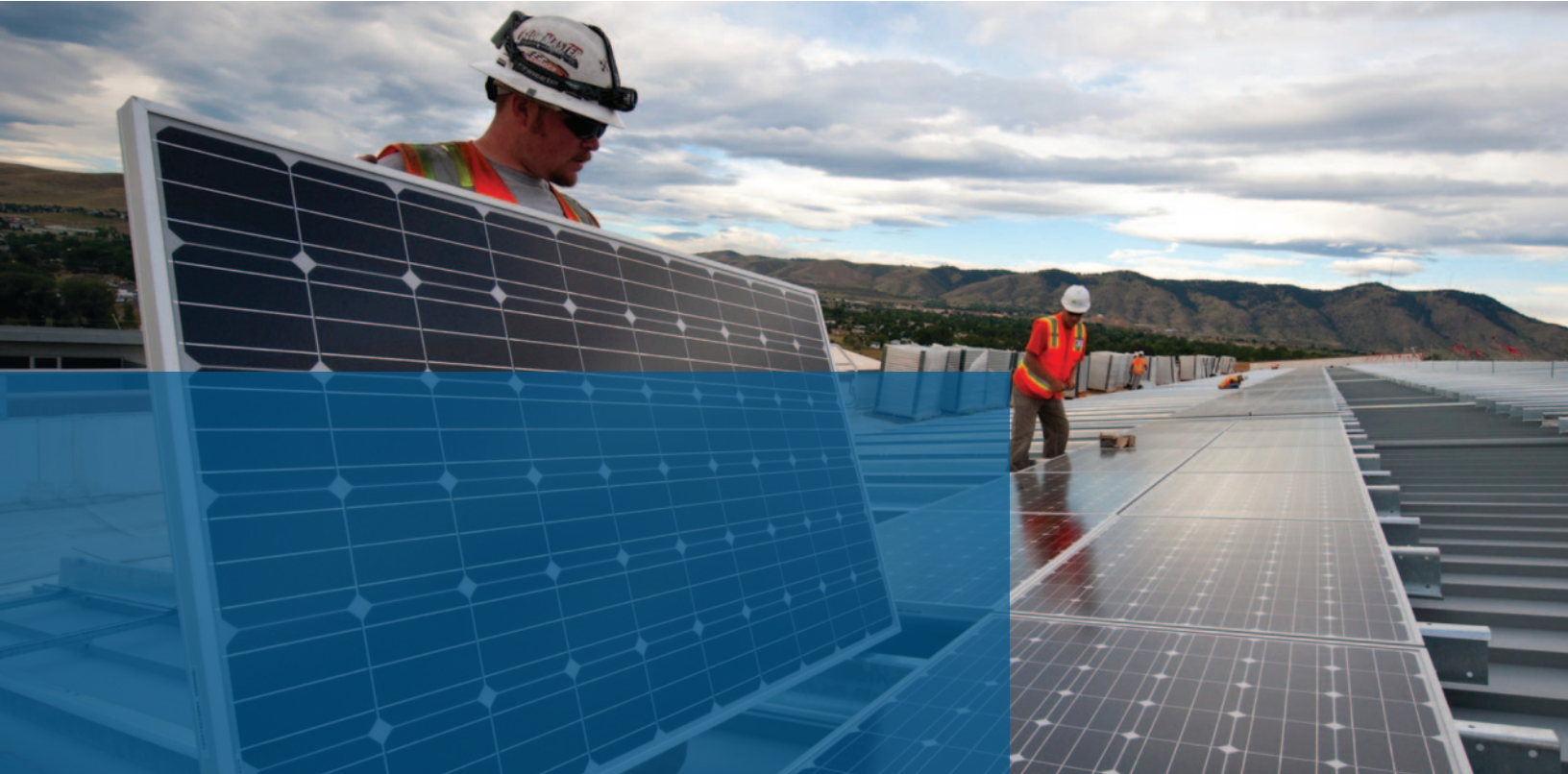
Installing solar energy, Rio de Janeiro Brazil. © Shutterstock/de freitas
