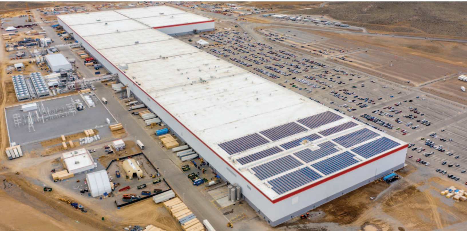
Tesla Gigafactory, Nevada, USA. © Shutterstock/Mizioznikov.
